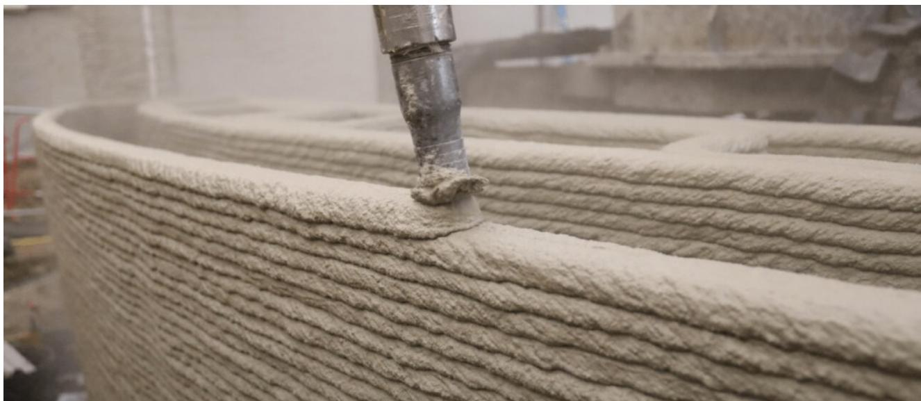
*Printing layers with the CyBe RC (Robot Crawler)*
