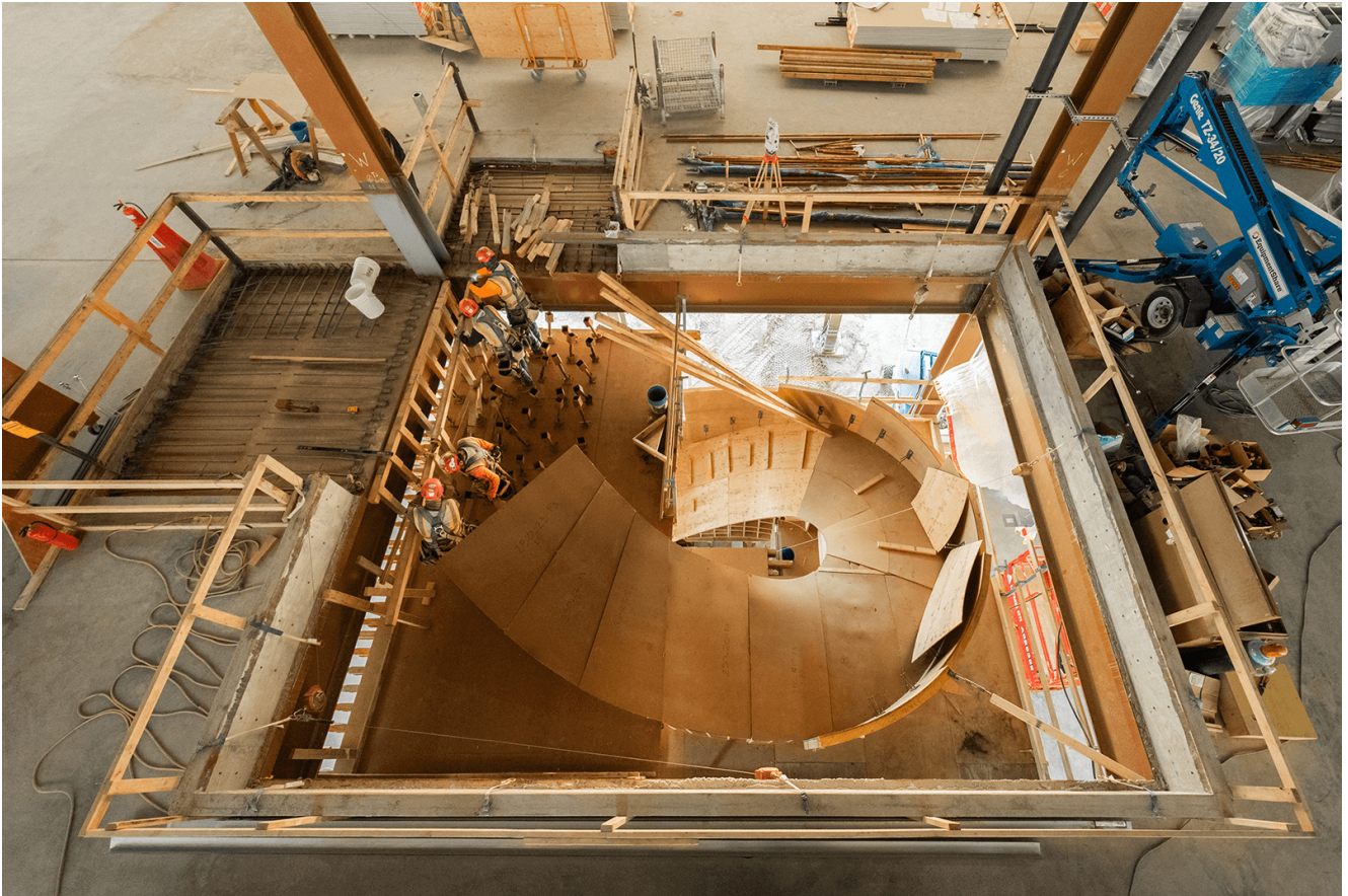
CNC-milled plywood formwork precisely captures the double-curved geometry defined in the computational model. Courtesy Clark Nexsen
