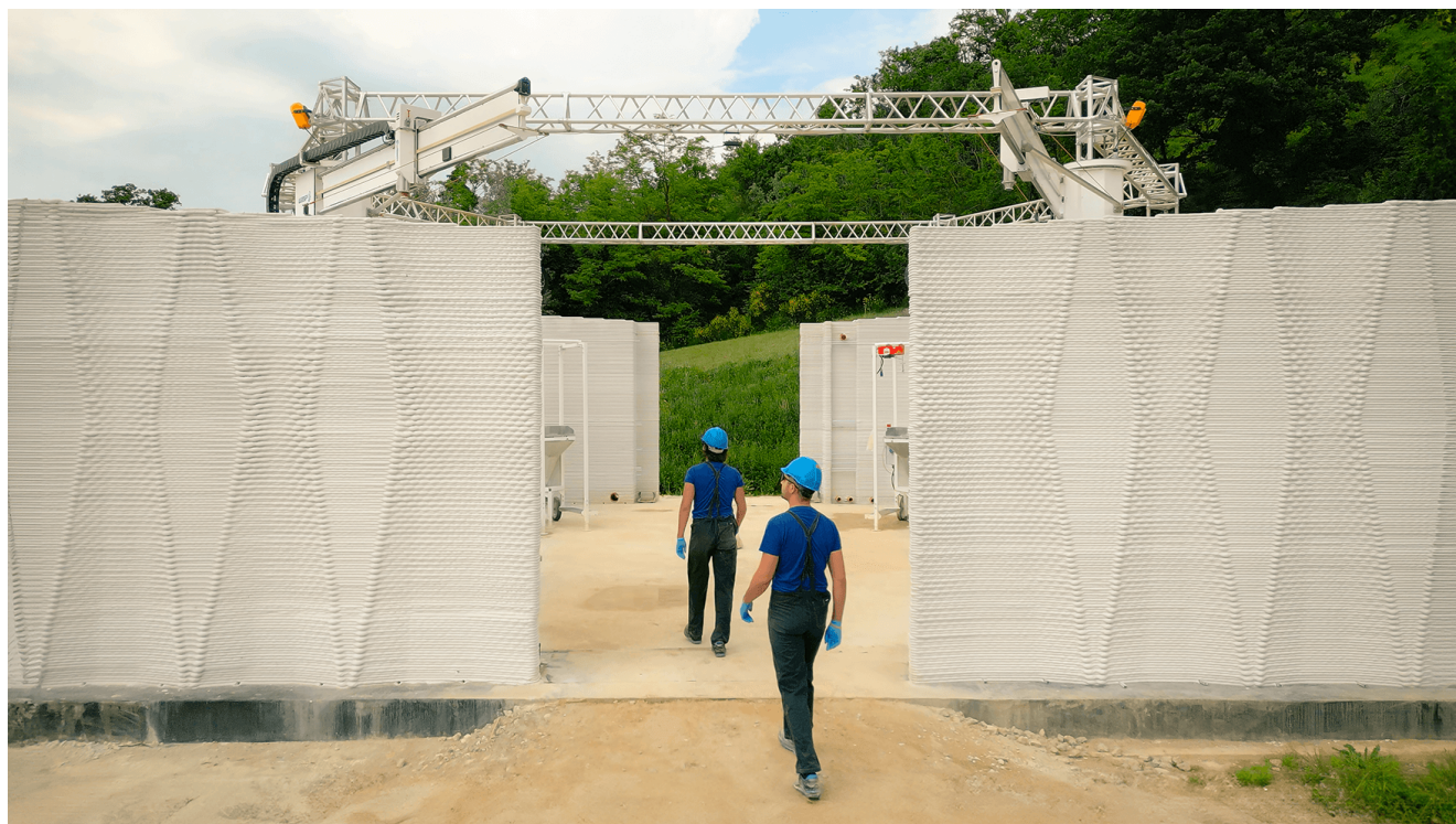
Completed 3D-printed walls forming the main entrance to the Itaca building during the construction phase.
