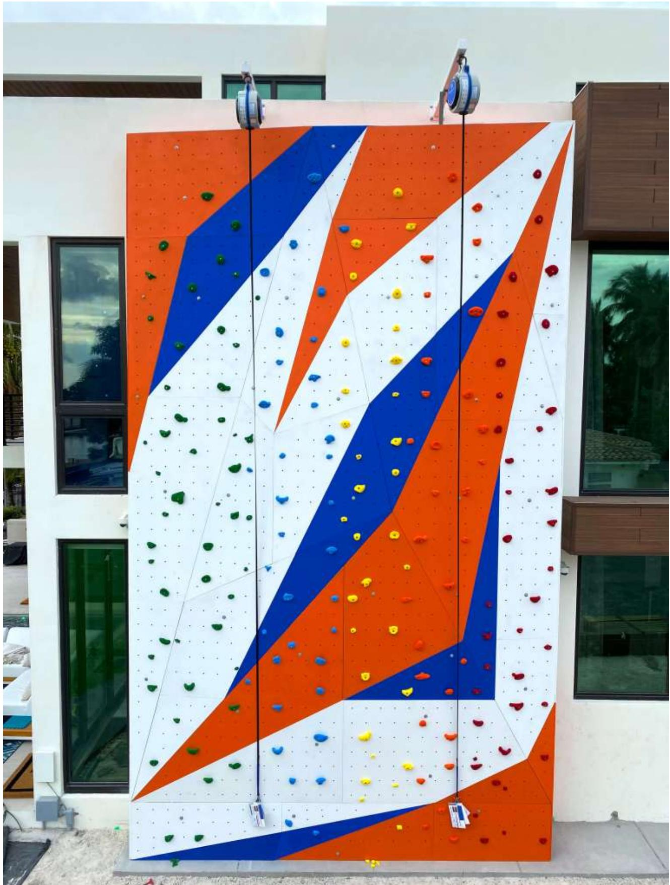
Precision during installation is a nonnegotiable goal. Each panel is a piece of the climbing wall puzzle, meticulously labeled and strategically reordered based on geometry. A grid of holes and extrusions cements the pieces together with unwavering alignment, a
