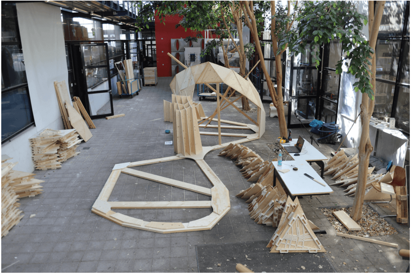
Early stage of pavilion assembly. The initial structural foundation and composite modules are positioned on-site according to the predefined assembly sequence, which was developed using augmented reality planning.
