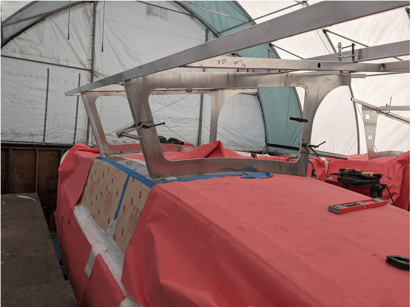
Aluminum superstructure under construction at ReVision Marine, translating the Rhino documentation into the physical vessel.
