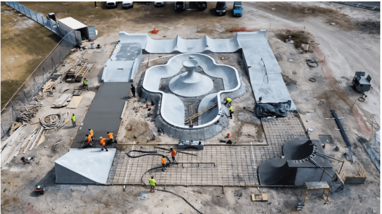
Drone view of the construction process.
